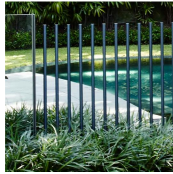
6 Metal Pole Balustrade 16MM ROUND METAL POWDER COATED: DULUX ELECTRO VENERABLE SILVER KINETIC
